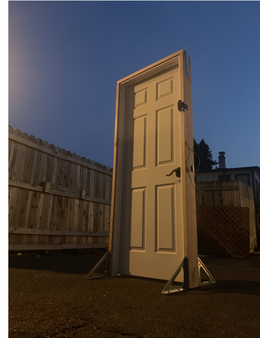
Figure 2: DOOR installation. Work in progress.
